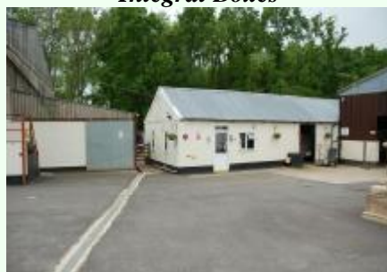
Yard view to Office
